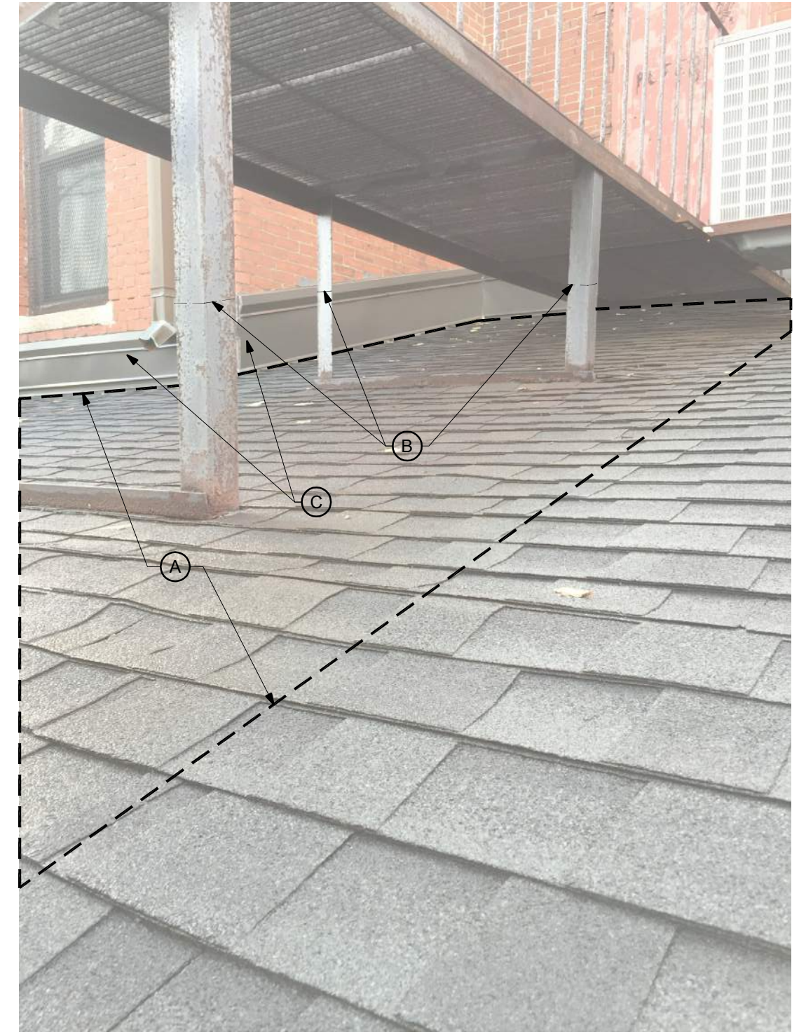
LOW ROOF DEMOLITION: ASPHALT SHINGLES TO BE REMOVED SCALE: N.T.S.
